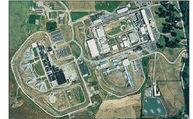
A bird's eye view of the Washington State Reformatory
